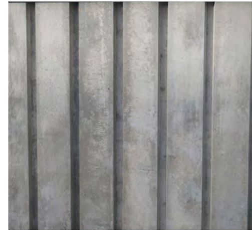
Betong sandwichvegg
